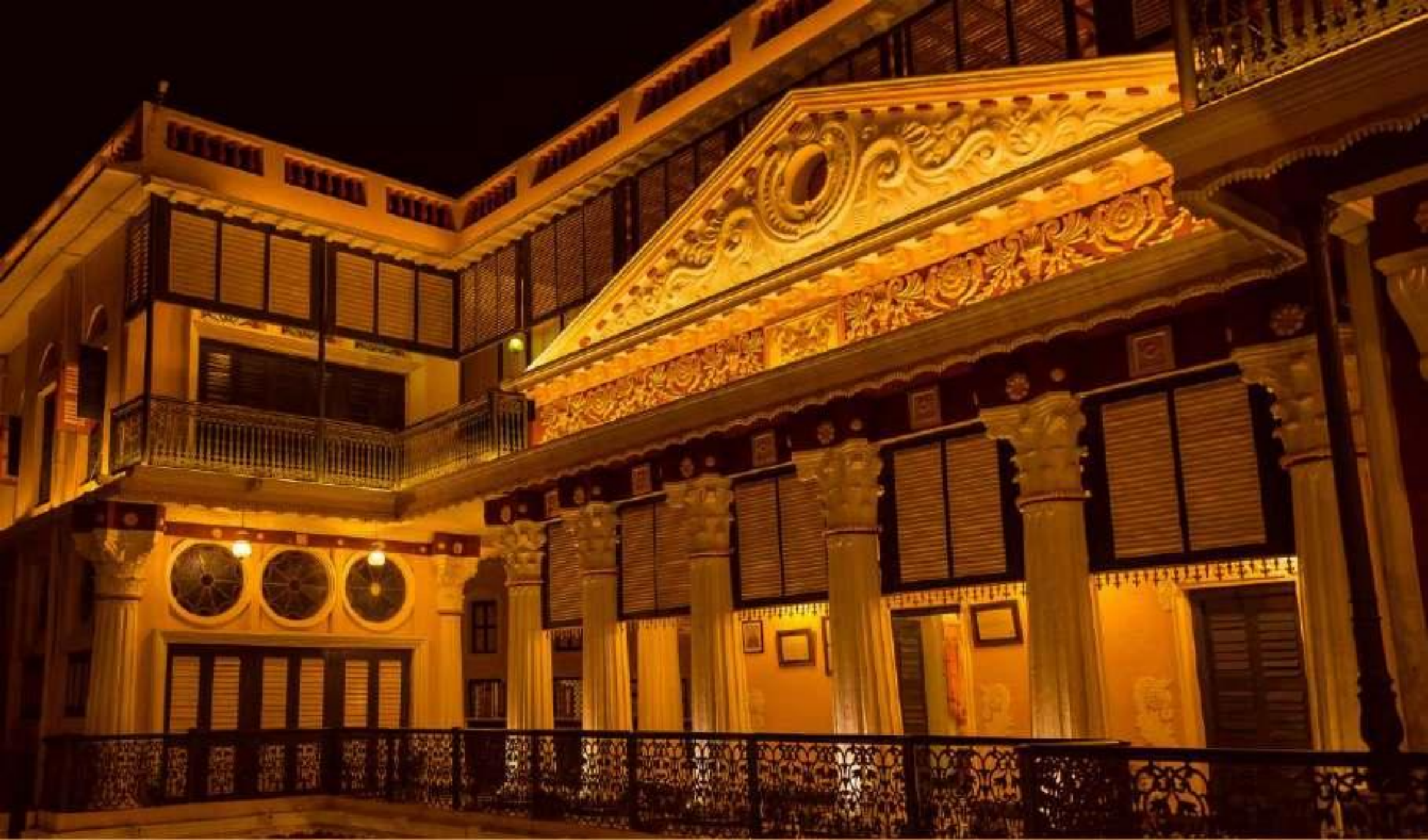
BARI KOTHI The First Heritage Hotel of Murshidabad
